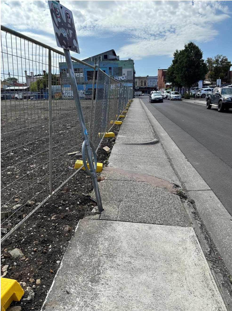
Figure 8: Subject site as viewed from Florence Street
