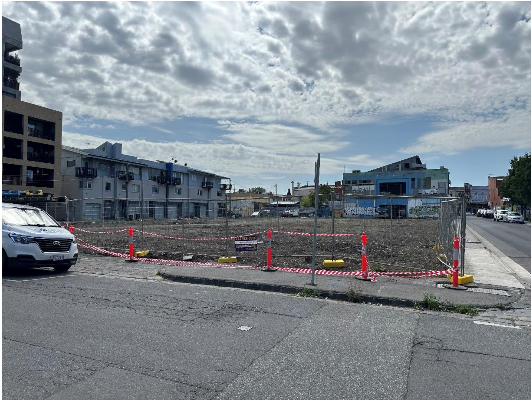
Figure 5: Subject site as viewed from Breese Street
